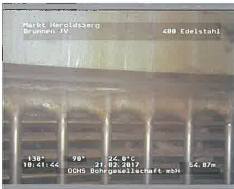
Foto: 104404_A.JPG, 00:05:59 54,87m, OK Filterrohr
