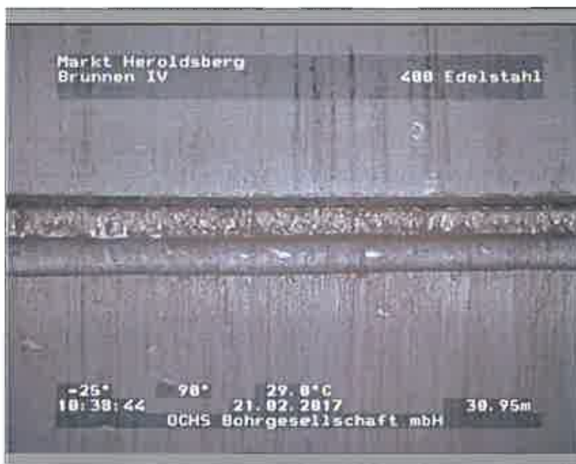
Foto: 104104_A.JPG, 00:03:04 30,95m, OK Vollrohr
