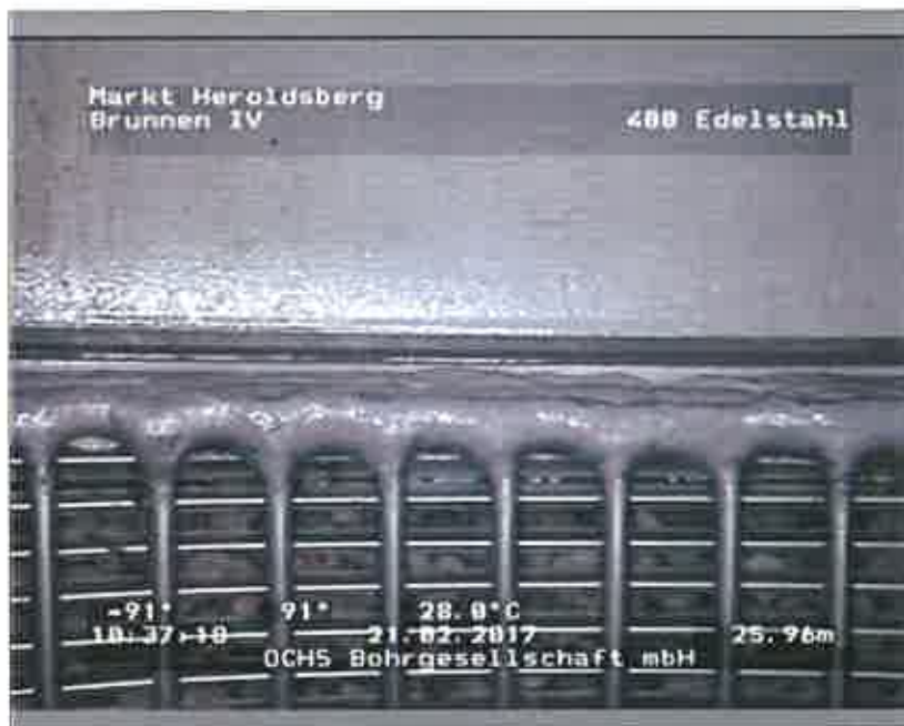
Foto: 103938_A.JPG, 00:01:52 25,96m, OK Filterrohr
