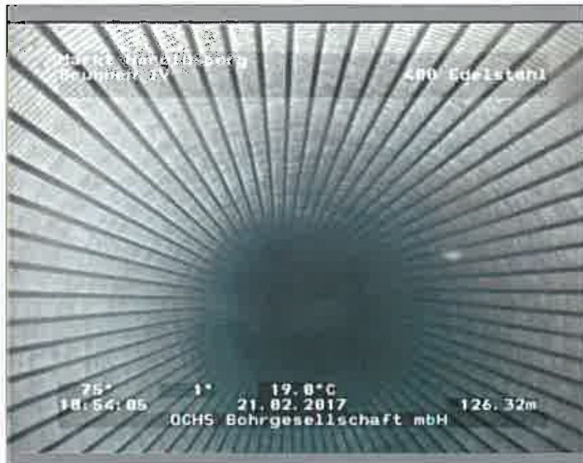
Foto: 105625_A.JPG, 00:17:44 126,32m, Blick ins Filterrohr, ablagerungsfrei
